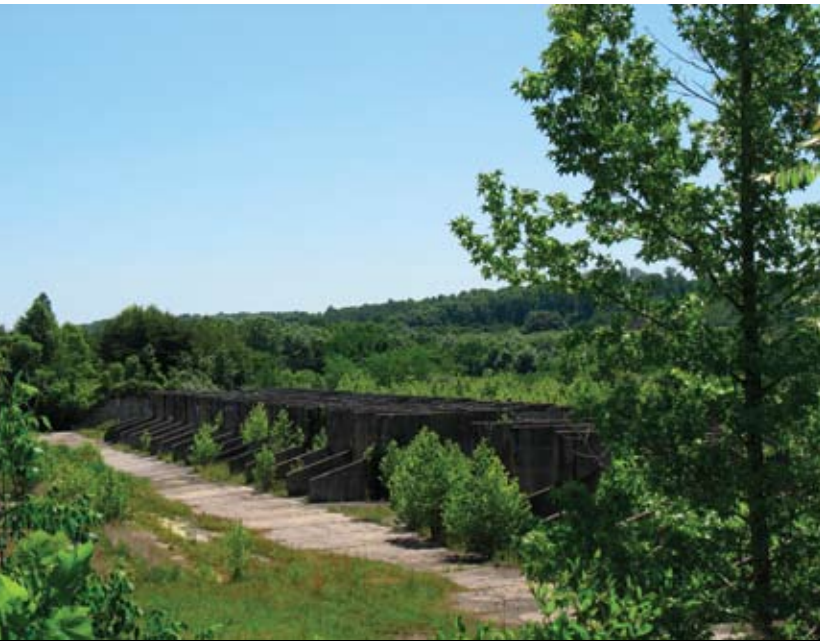
Project: Former Chrome Foundry Location: Tennessee Client: Confidential
