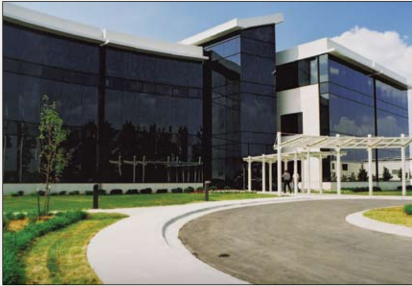
The award-winning Bayer Central Administration Facility, Shawnee, Kan., features 50,000 square feet of offices, conference rooms and cafeteria facilities.
