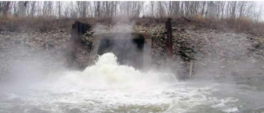
Heated discharges can be disruptive to cold-blooded organisms that live in water. Facilities can receive a variance from water quality standards regulating the temperature of discharges through Section 316(a) of the Clean Water Act if they can show the receiving water body is maintaining a balanced, indigenous aquatic community.
