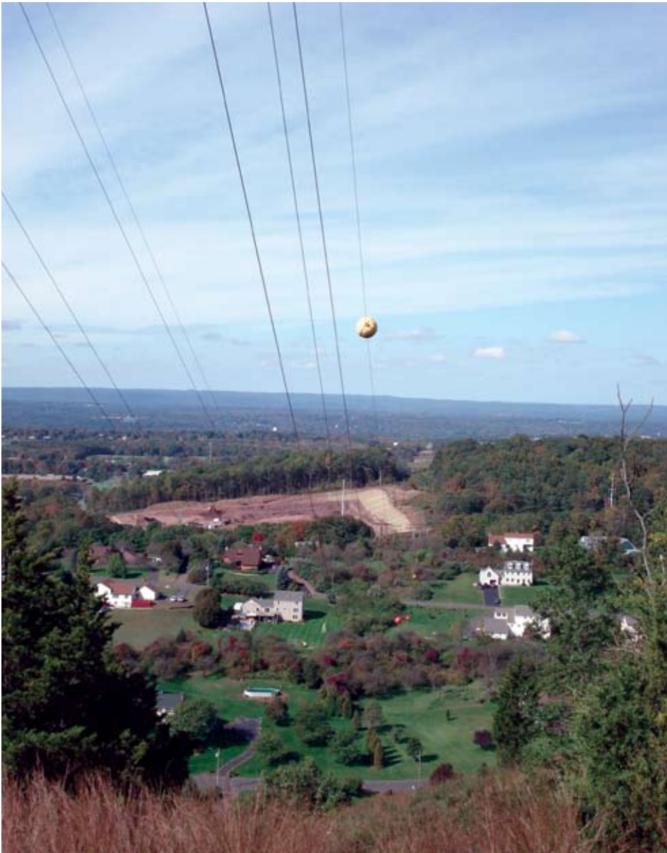
The view from Beseck Mountain of the cleared site for the new Beseck Switching Station in Wallingford, Conn.
