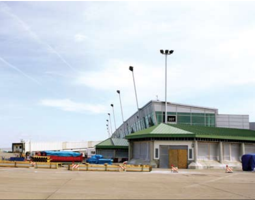
Project: Airport Security Upgrades Location: St. Louis Client: Lambert-St. Louis International Airport
