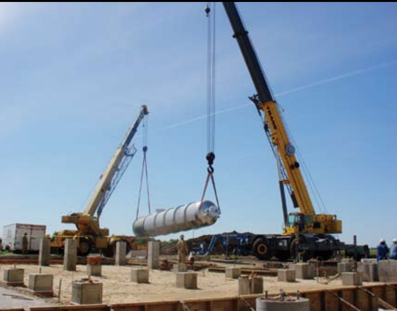
Project: Natural Gas Plant Renovation Location: Bushton, Kan. Client: ONEOK
