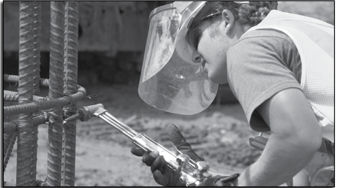
Figure 2 : After a field redesign, a foundation crew member prepares to cut off a rebar cage to shorten it as required.
