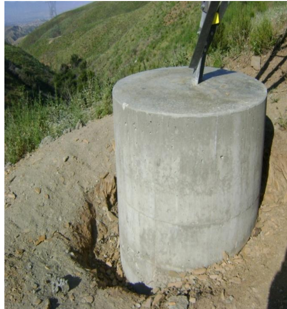
Figure 5: A complete micropile foundation is indistinguishable from other types on the surface.
