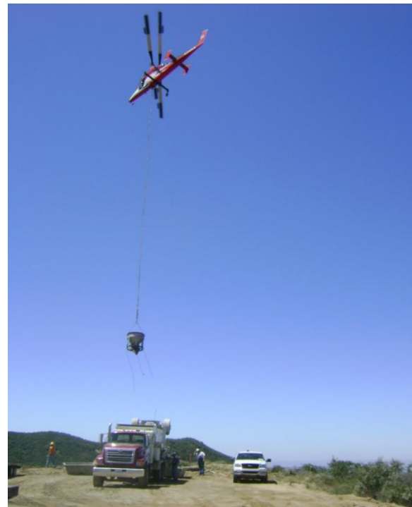
Figure 12: A K-Max helicopter transports volumetric concrete to the tower site.
