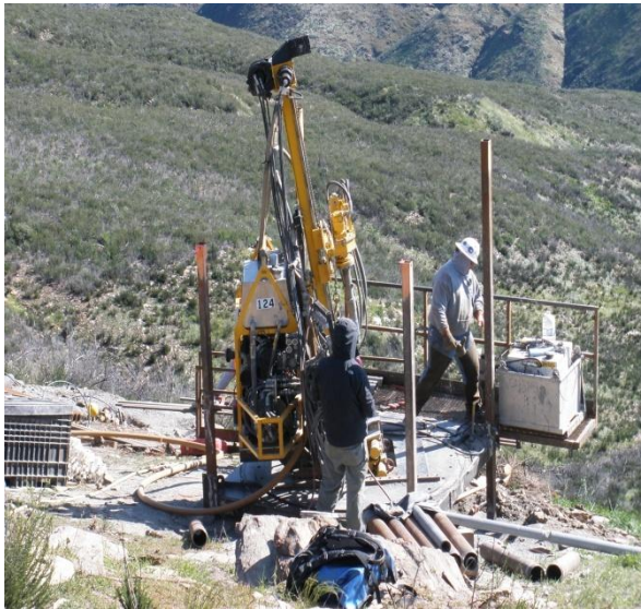
Figure 9: Micropile drill platform and drill rig.
