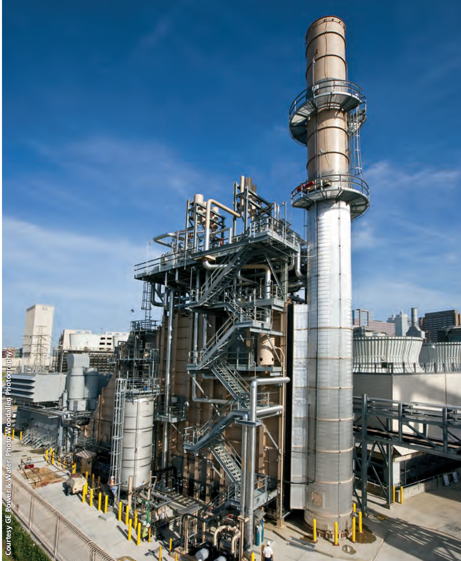
The heat recovery steam generator is a key component of TECO's on-site CHP system, which recovers waste heat via conductive heat transfer to produce steam.
