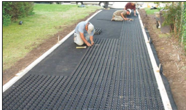
Figure 2-1 Grass and Gravel Pavers Installation
