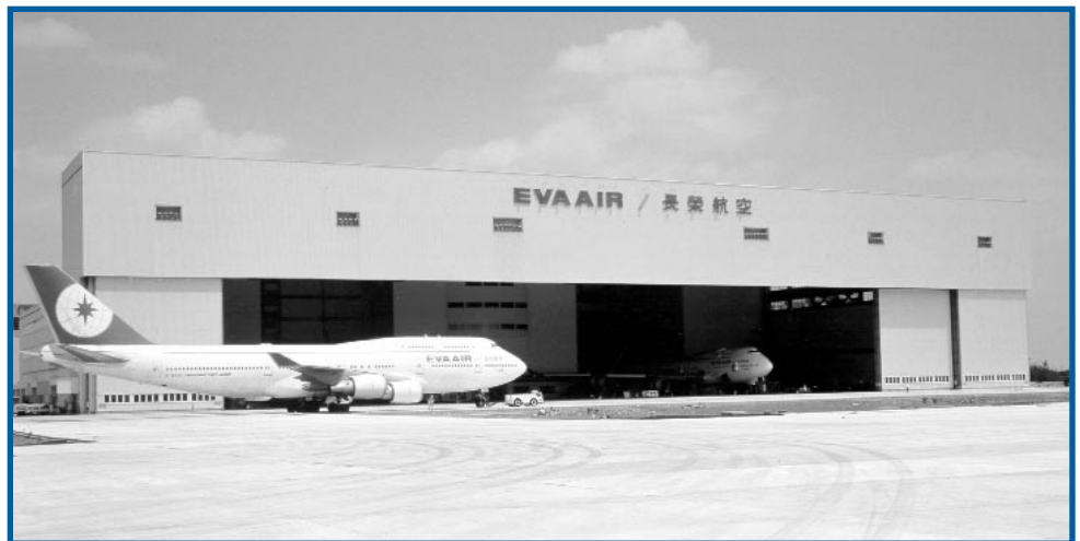
160-meter clear-span aircraft maintenance facility for Evergreen Airways in Taiwan, Republic of China. This structure utilizes a space frame roof system with a lateral load resisting system composed of braced frames.
