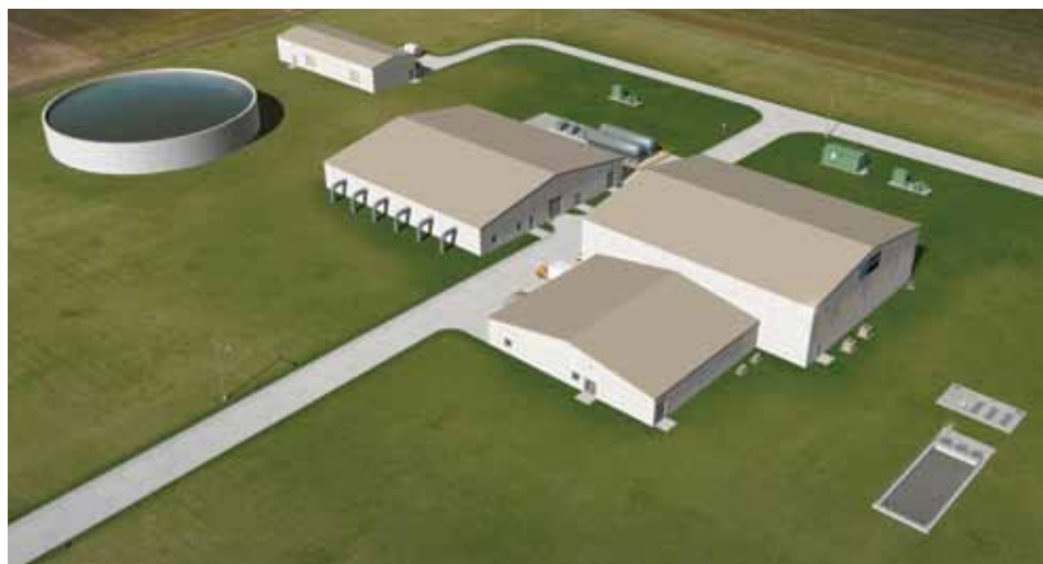
Water drawn from the Little Arkansas River during high flows is treated and pumped into the Equus Beds Aquifer, where it is stored and later recovered.
