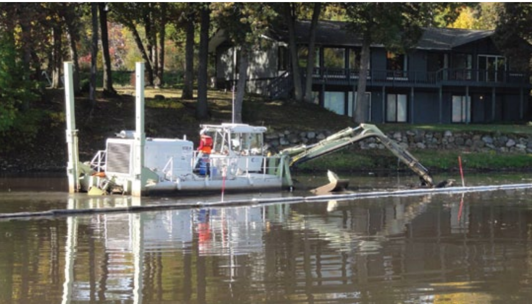
Workers dredge the Kalamazoo River above the Ceresco Dam.
