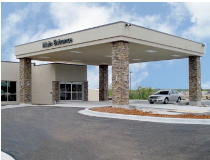
Walden Structures, a California company, fabricated the modular structure for the interim 150,000-square-foot hospital that was transported from California and erected across from the old site.
