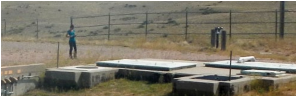
Jennifer Ross looks over surface access to an underground launcher equipment building (LEB) near F.E. Warren Air Force Base in Wyoming. Filling the cavity of a single LEB will require 346 tons of sand, rock or other aggregate.
