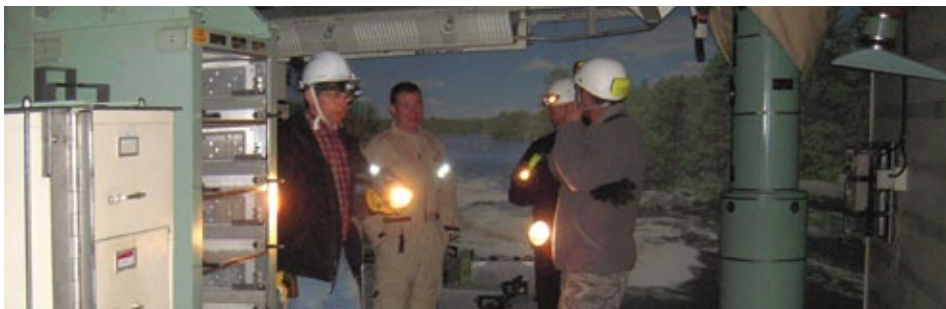
At missile facilities — including this one in Montana — to be filled and then covered with concrete, below-ground inspections will be history. “The cap is going to be there forever,” Jennifer Ross says.
