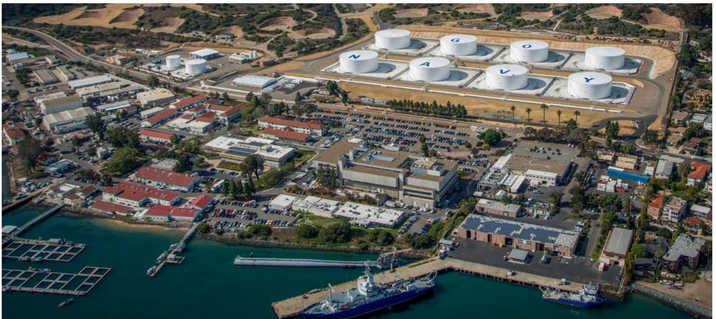
The eight new storage tanks occupy a smaller site than the tanks they replaced, while maintaining a storage capacity of 1 million barrels at the Point Loma NAVSUP FLC San Diego.
