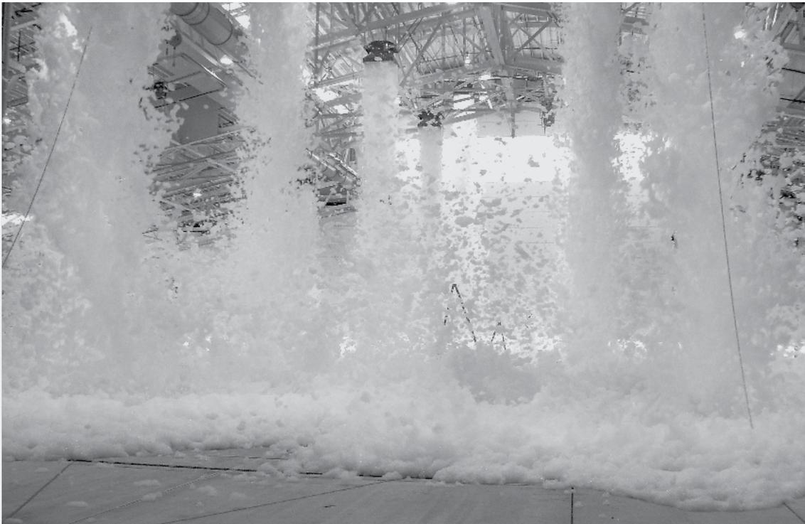
Image 2: High-expansion foam has become a preferred option for fire suppression in large, open facilities such as aircraft hangars.
