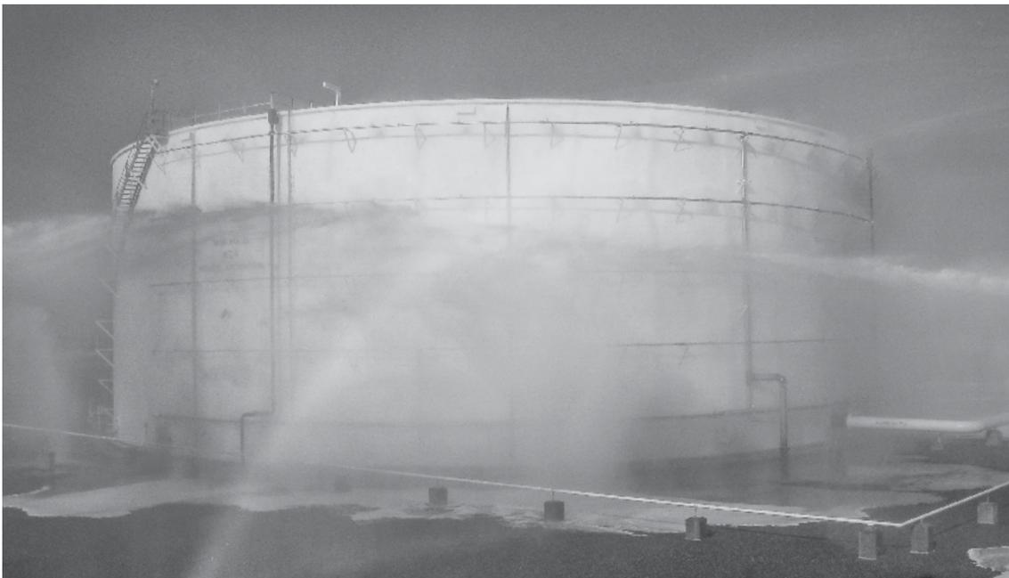
Image 1: A hydrocarbon product storage tank uses an exterior water spray system for cooling, internal protection via foam (AFFF) chambers and dike area protection with high-volume foam/water monitors.
