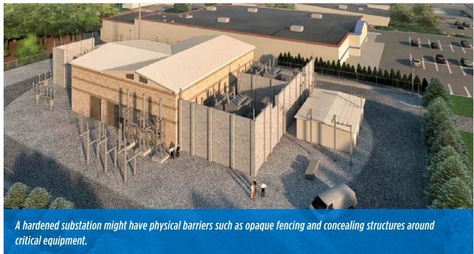
*A hardened substation might have physical barriers such as opaque fencing and concealing structures around critical equipment.*
